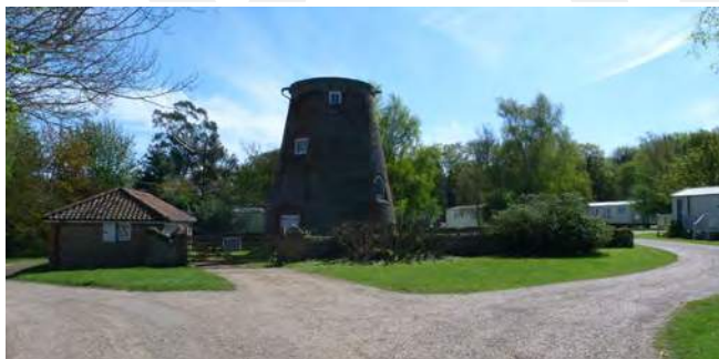
The former mill within the caravan site
