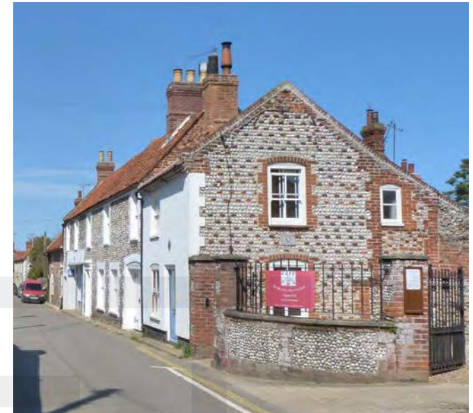
Brick and flint used in decorative patterns on a house on the High Street
