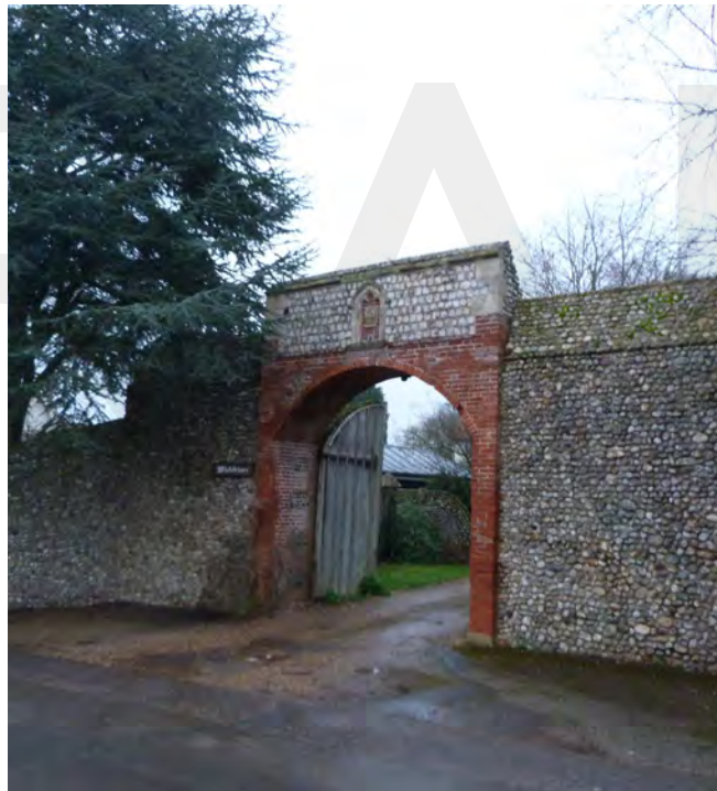
Listed friary gateway and wall at the north end of Back Lane, with sloped flint capping detail
